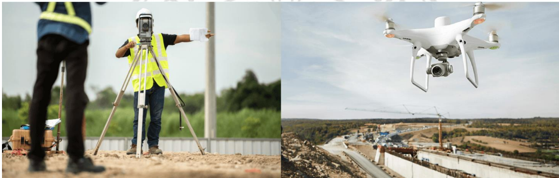
Figure 2 Technology for data collection; ground-based methods (left), and aerial-based method (right) (Heliguy, 2022).
