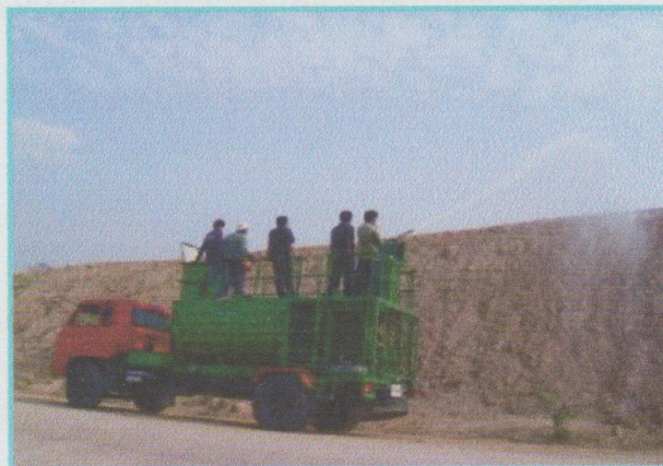
Figure 1 Hydroseeding
