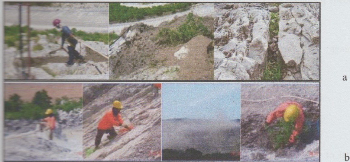
Figure 3 Methods of reclamation mines by SCG a) Mud Slurry Seeding Method b) Blow up Soil for Plant Method
