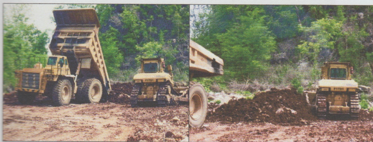
Figure 2 Typical grading and tracking-in operations for non-forest post mining land use
