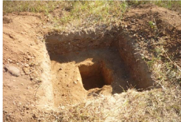
Preparing a pit trench
