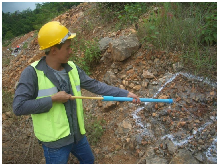
Hydroseeding application at limestone mine by PVC water pistol.
