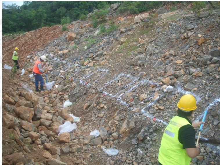
Plots on a slope at limestone mine.
