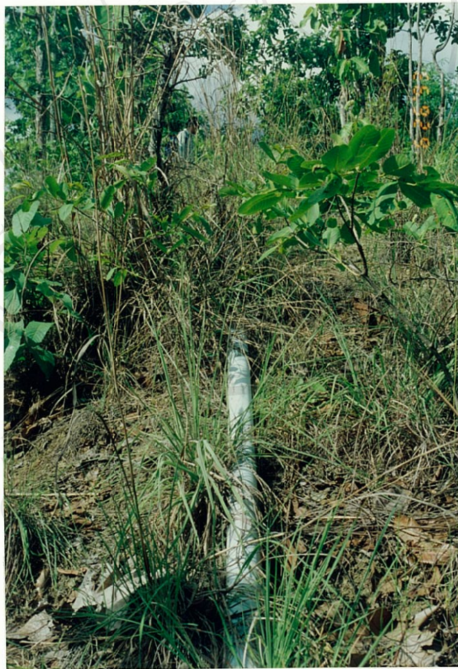
Figure 2. Pipes laid along the ridge of the irrigated area.
